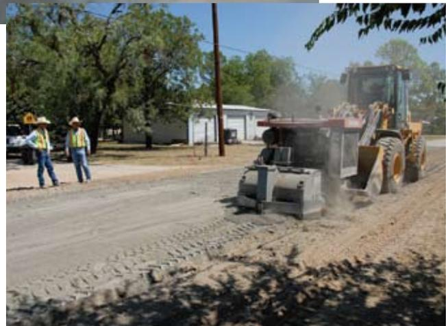
inches of the existing asphalt, base and native soil, and 27 pounds of Cem-Lime per square yard or about 3/4 inch spread evenly over the surface of the road.
