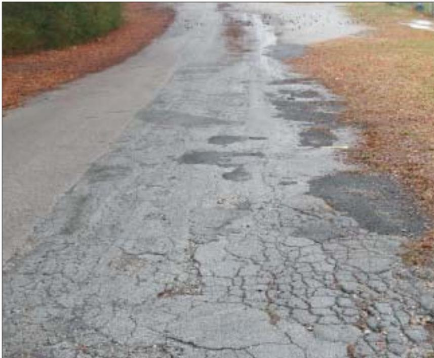
*The roadway and parking areas surrounding Hixson Ball Fields evidenced severe distress and poor drainage.*
