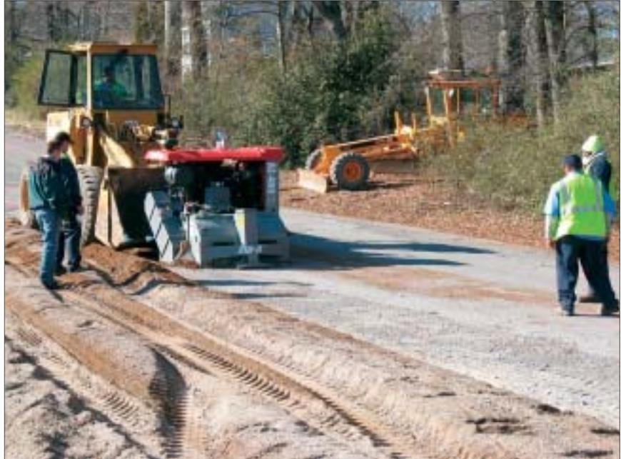
*The pavement reclaimer pulverizes the existing pavement structure to a predetermined depth. The resulting material is graded and compacted in-place to form a new base or subbase.*
