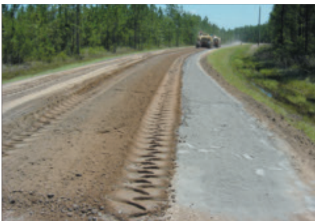
FDR with cement recycles existing asphalt pavements and aggregate bases to create a thicker pavement structure and a longer lasting base.
