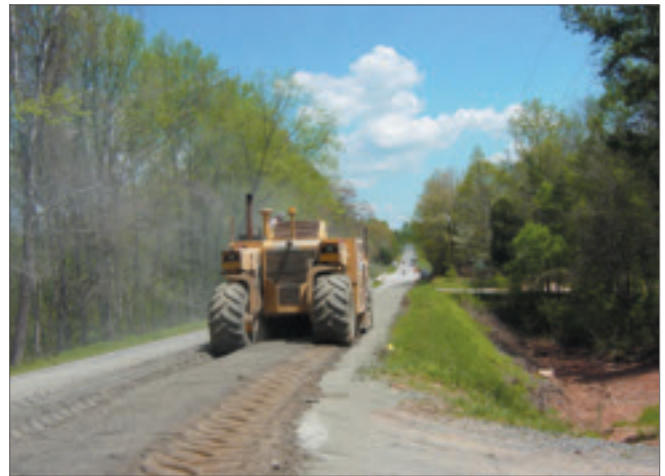
Full-depth reclamation using cement can cut costs up to 50 percent and will increase the longevity of roads.
