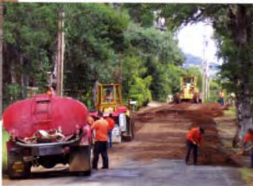
Lake County (California) uses its Asphalt Zipper unit both for road patching and, occasionally, to recycle an entire roadway (left). Below, Lake County Crews performing FDR for road reconstruction.
