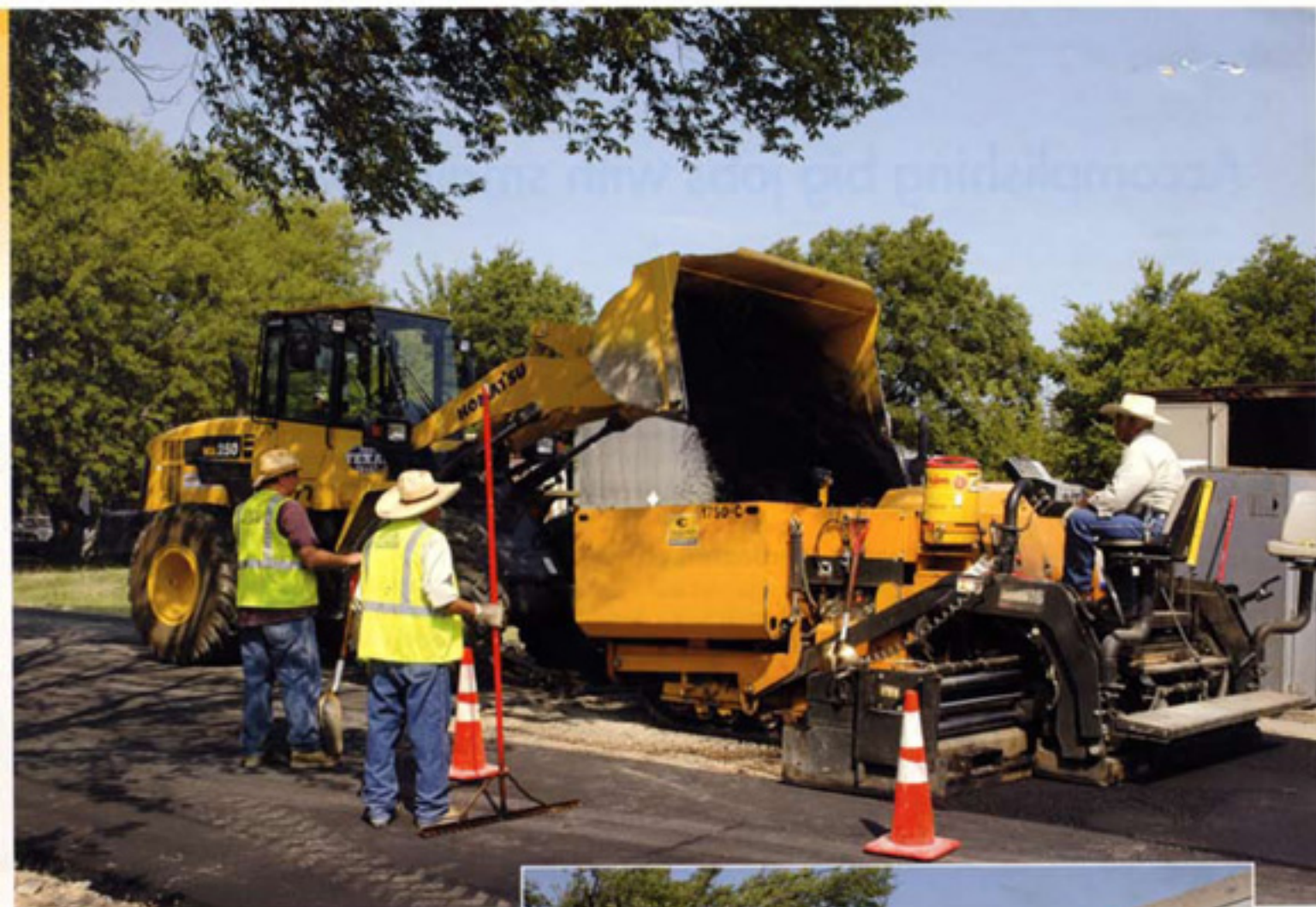
(Right) Mauricio Abrego with the city of Hillsboro takes on a load of asphalt mix with the Komatsu WA250-6 wheel loader, which he then uses to feed the city's asphalt paver (above).
